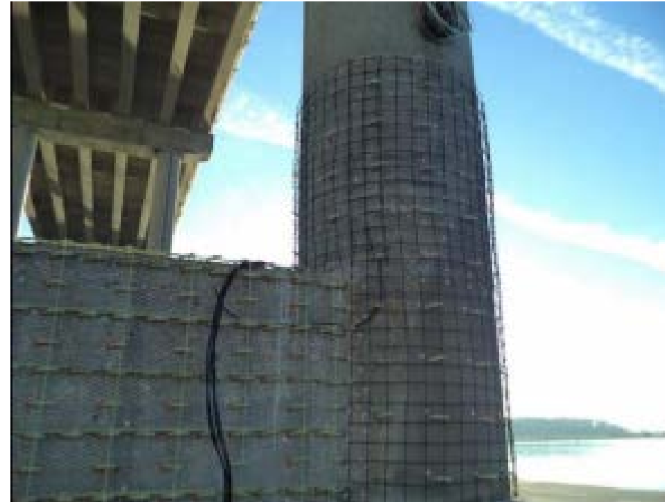
FDOT Bridge Substructure Rehabilitation
