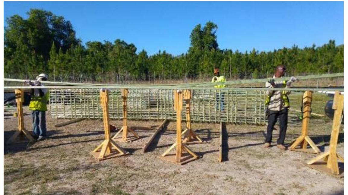
Construction Crew Lifting Reinforcement Cage.
