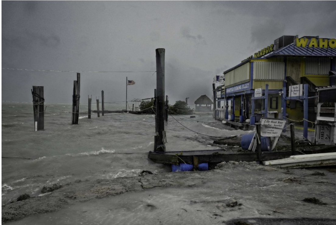
Dock Damaged by Hurricane Irma in Islamorada, FL.
