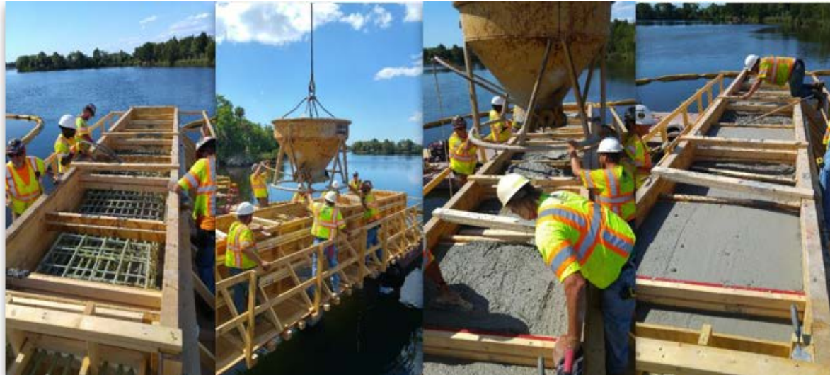
FDOT Bridge Rehabilitation project. GFRP and CFRP Used in Concrete Deck
